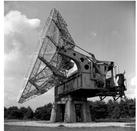
The Wurzburg Riese Antenna at Radio Kootwijk in The Netherlands that was used to confirm the detection of the 21 cm hydrogen line. Lex Muller is seen descending the stairs. (<http://wiki.waarnemen.com/index.php?title=Bestand:Wurzburg.jpg>)
